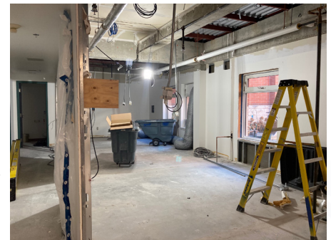
construction inside visitation space
